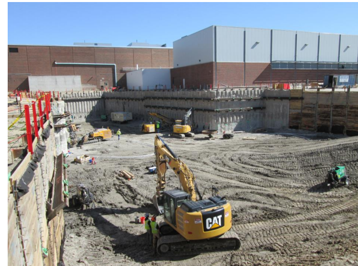
Excavation on west end of site
