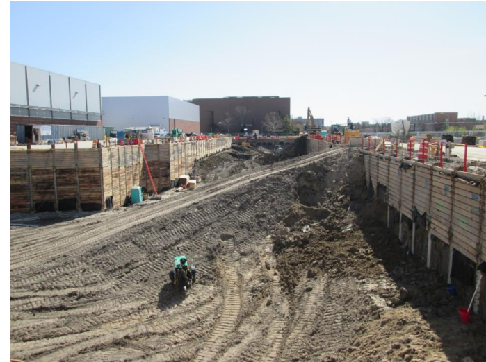
Excavation for linac tunnel
