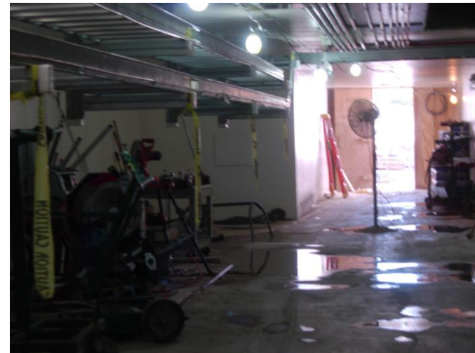
Tunnel View of Diagnostic Absorber after surrounded in concrete
