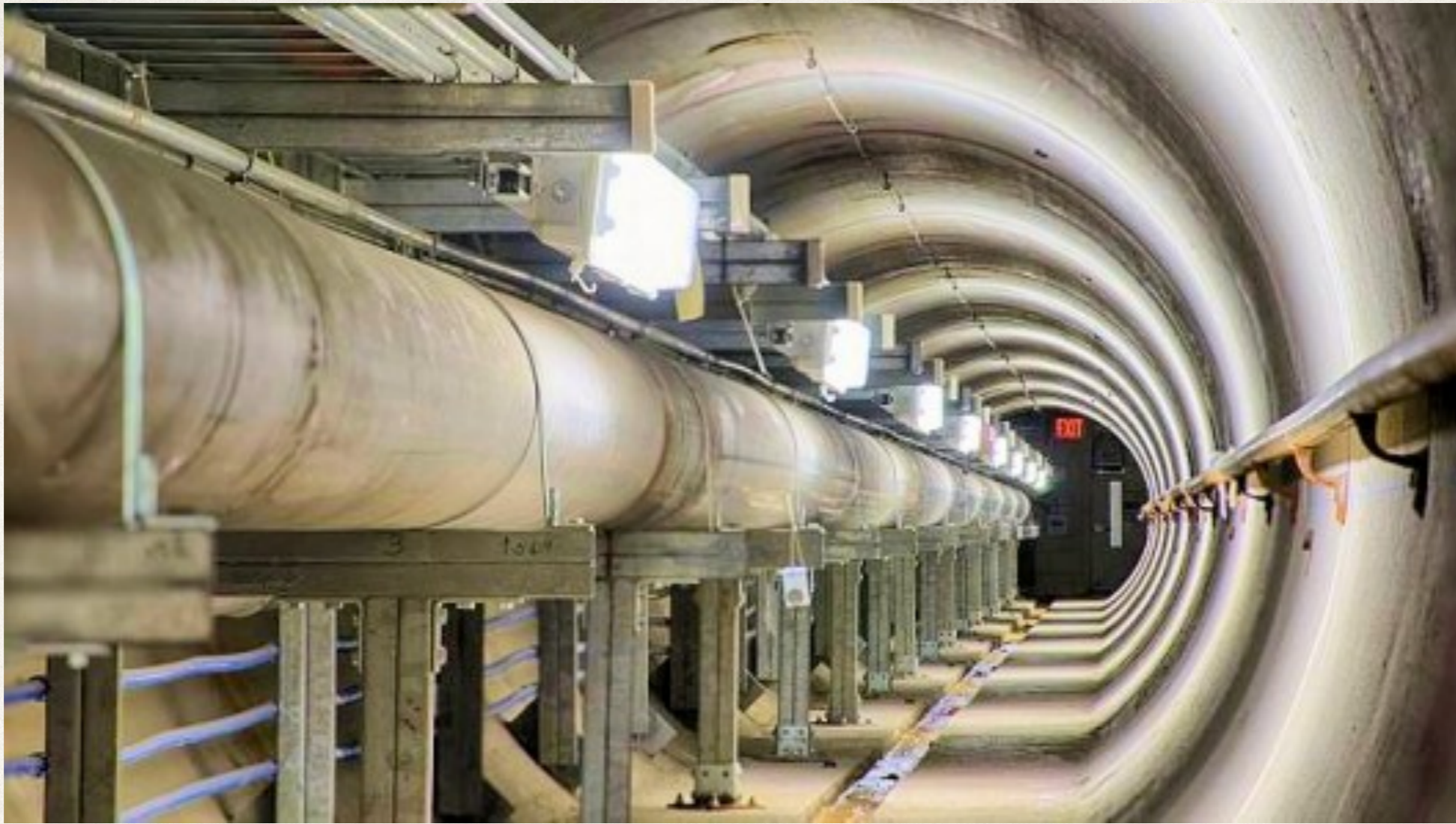
FNAL Main Injector Tunnel
