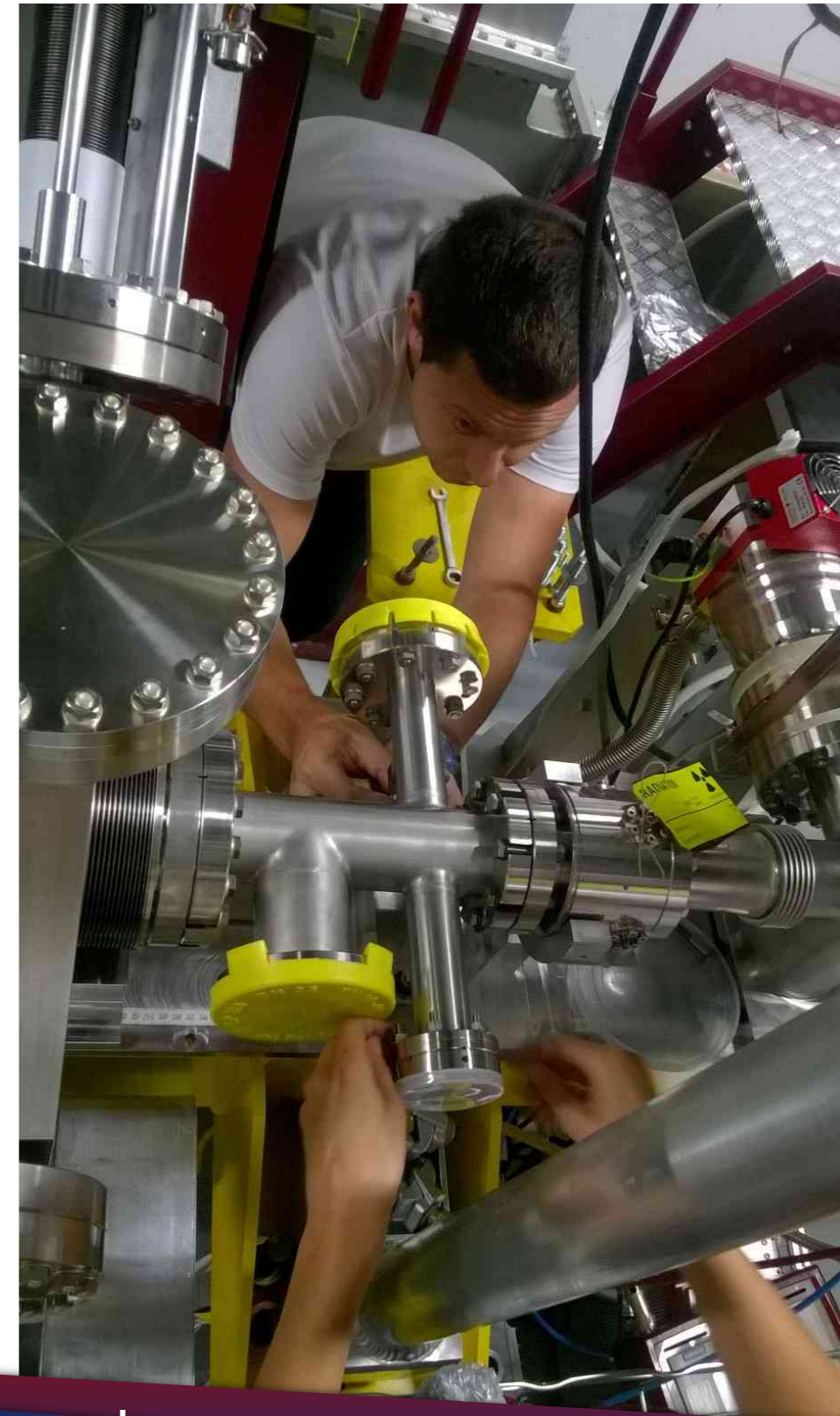
Vacuum chamber installation in Linac4
