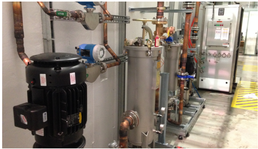
Pumps outside cave
