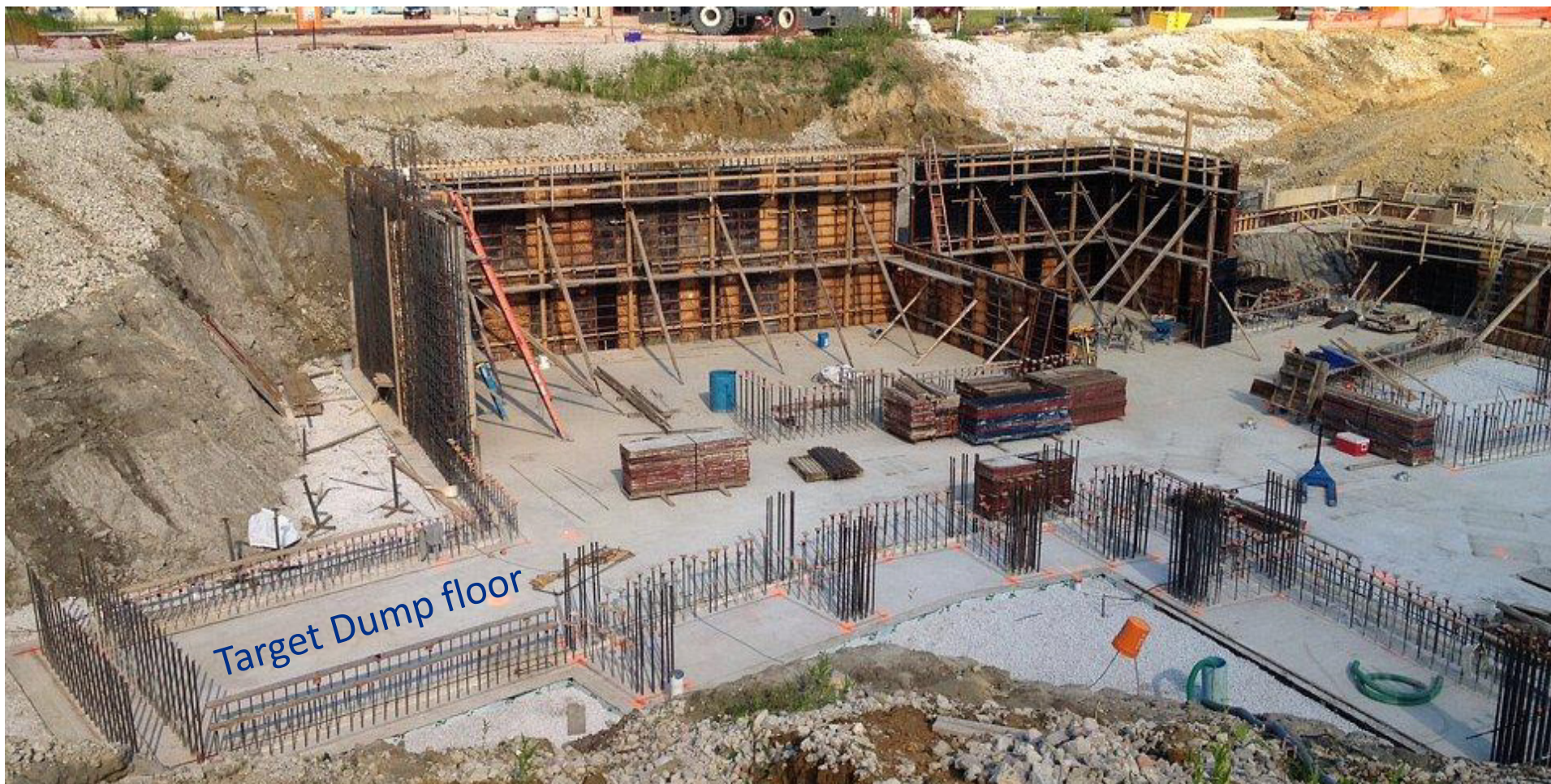
Framing the walls in the proton target station area of the Mu2e building
