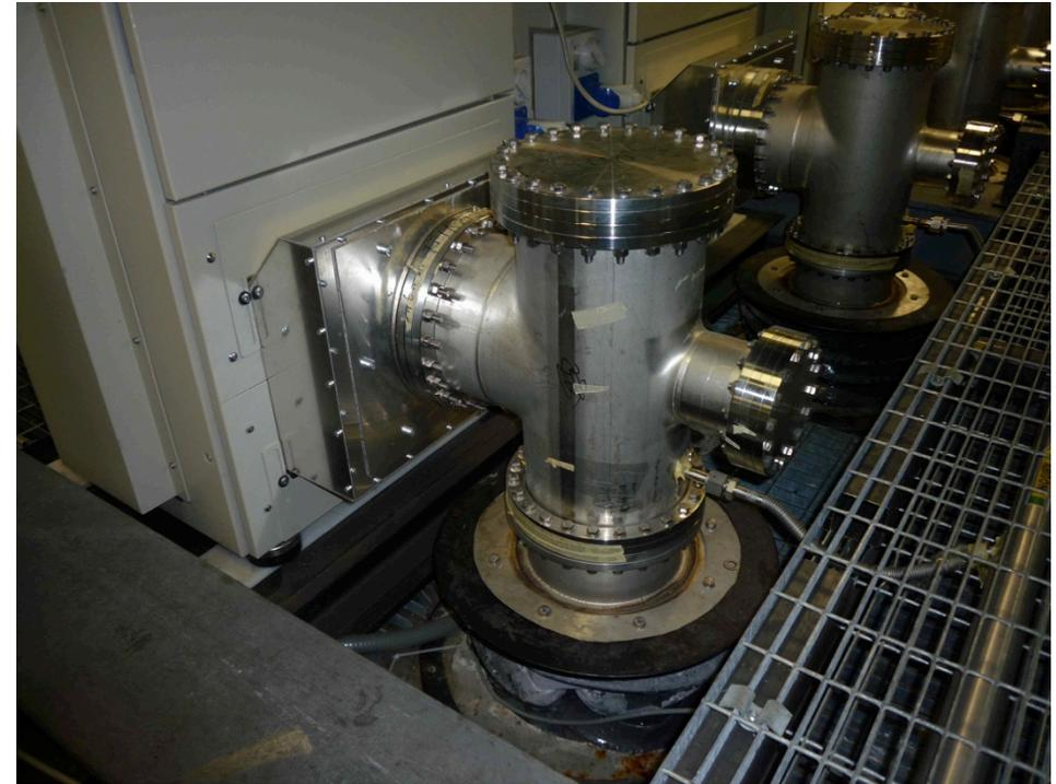
Signal flanges are connected to the back of the racks with a metal screen shielding twisted pair cables.
