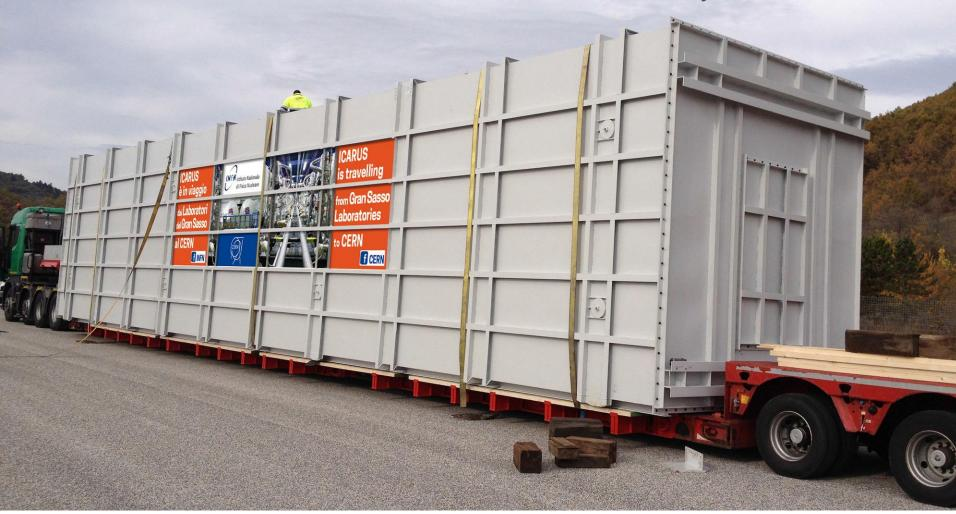
The rigging contractor will lift the T300 off the trailer and place it on track rollers so it can be rolled into the building. Fermilab personnel does the rest of the installation work.
