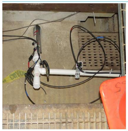
Sucks water from drain through sediment settlement system with pneumatic diaphragm pump. Pump can be turned off remotely for vinegar injection.
