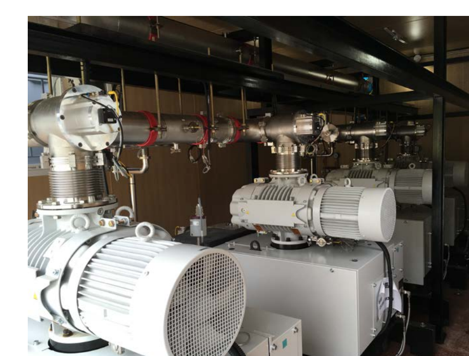
Warm pumps for superfluid helium
