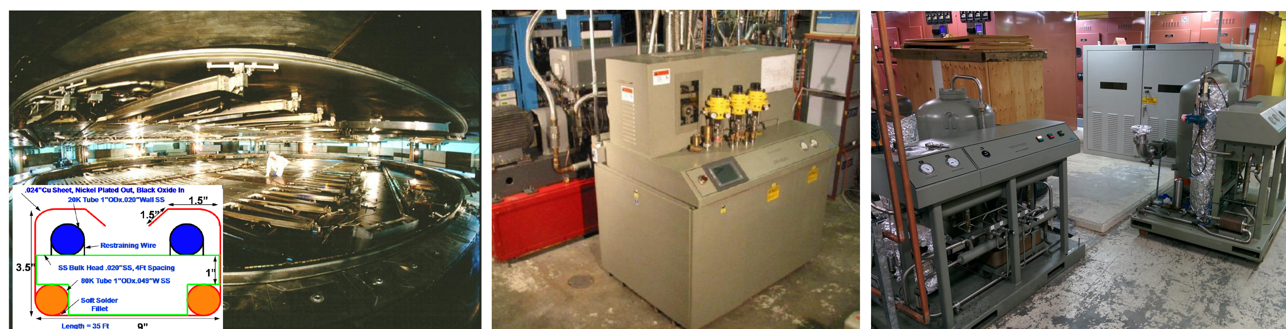
Cyclotron tank, Linde 1630 helium refrigerator, operational and spare compressors
