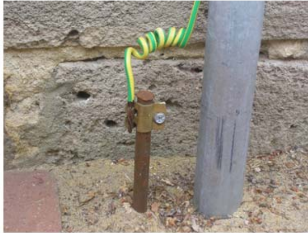
Figure 1.4.1. Left: Earth Ground Symbol. Right: Earth Ground Rod. Image courtesy of Wikipedia: https://en.wikipedia.org/wiki/Ground_(electricity)
