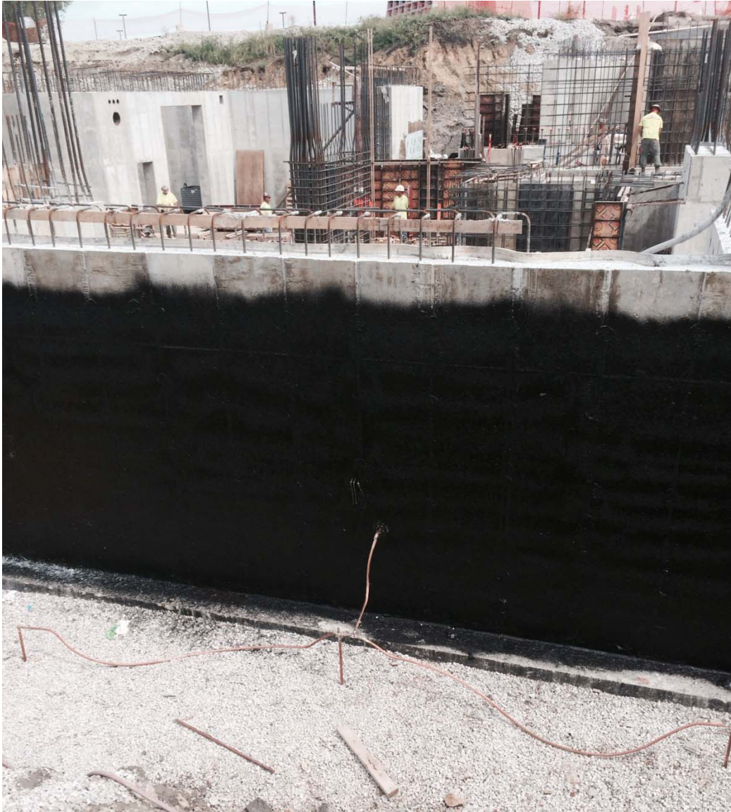
Figure 4.9.4. Implementation of one of the Detector Ground networks.
