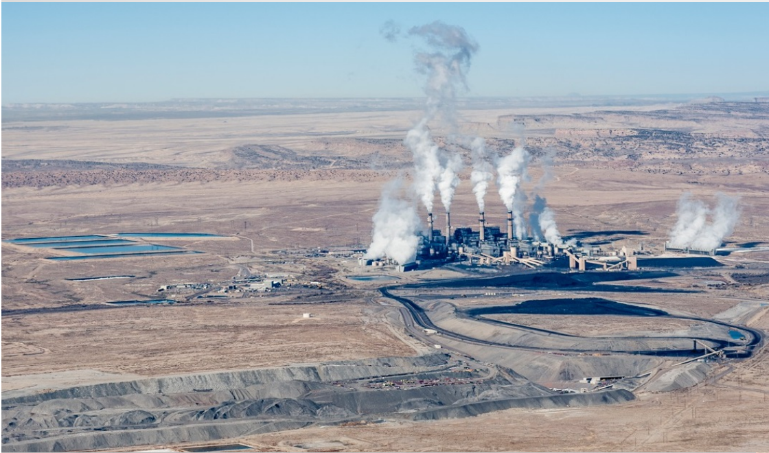
Four Corners coal-fired power plant
