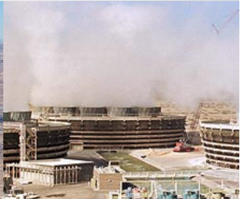
Cooling towers at Palo Verde nuclear plant near Phoenix, AZ
