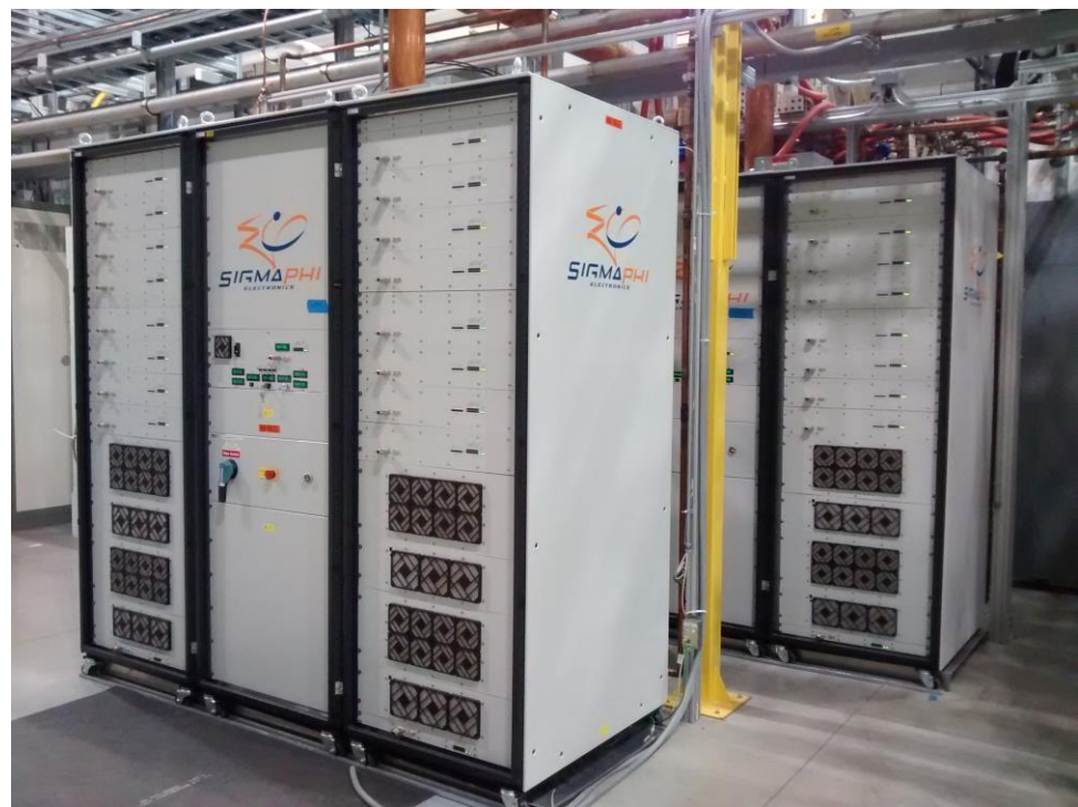
SigmaPhi 162.5 MHz 75 kW Amplifiers
