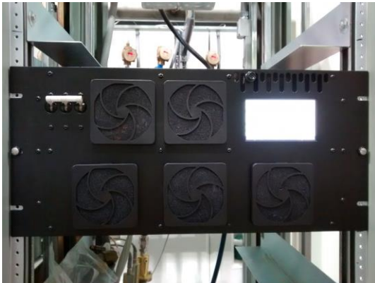
Comark/Technalogix 3 kW amplifier
