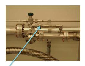
Nitrogen in-line and point of use filters: Mott Defender series sintered all metal (0.03 micron)
