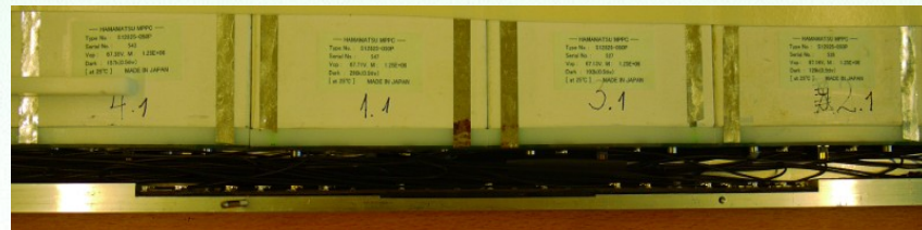
32 coax cables inside
