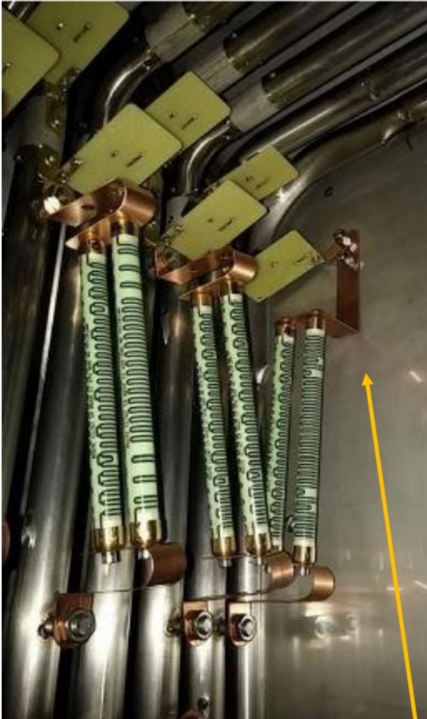
Detail – attachment of resistor chain to the cathode
