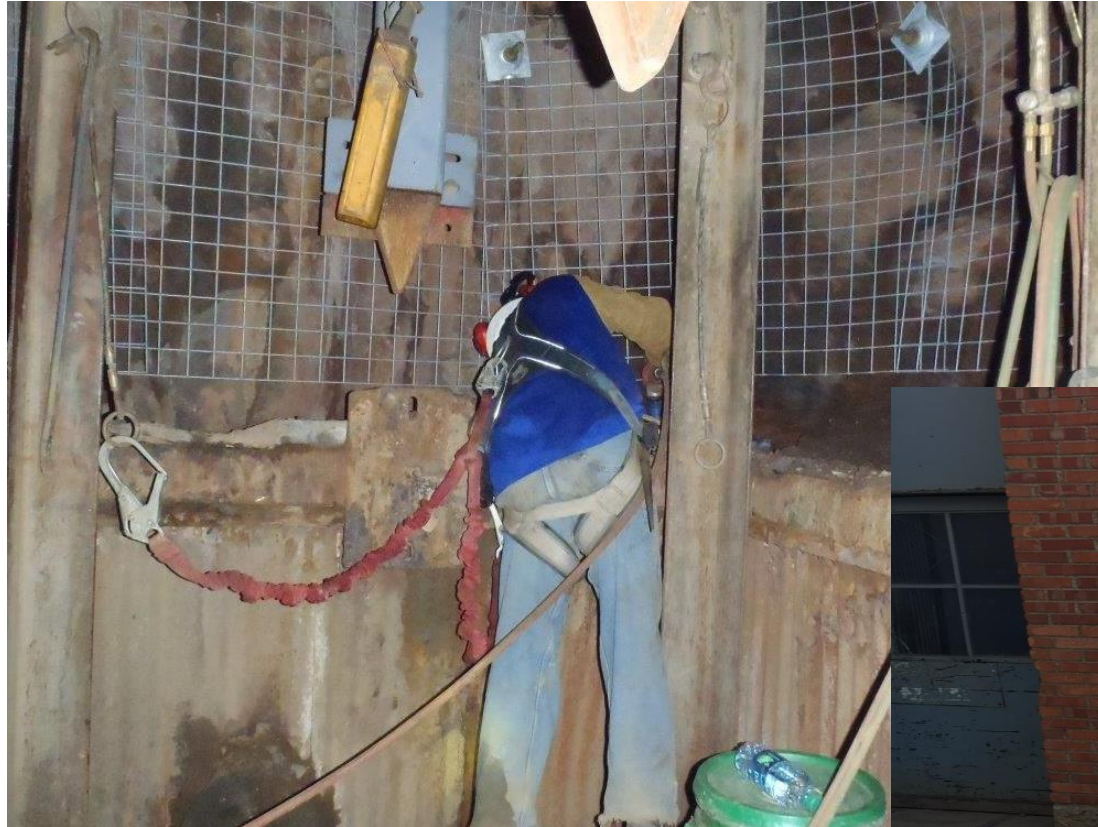
Removing old set
