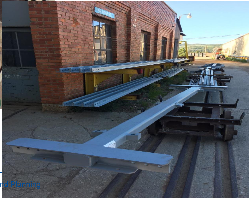
Steel set 280 staged & ready to be installed
