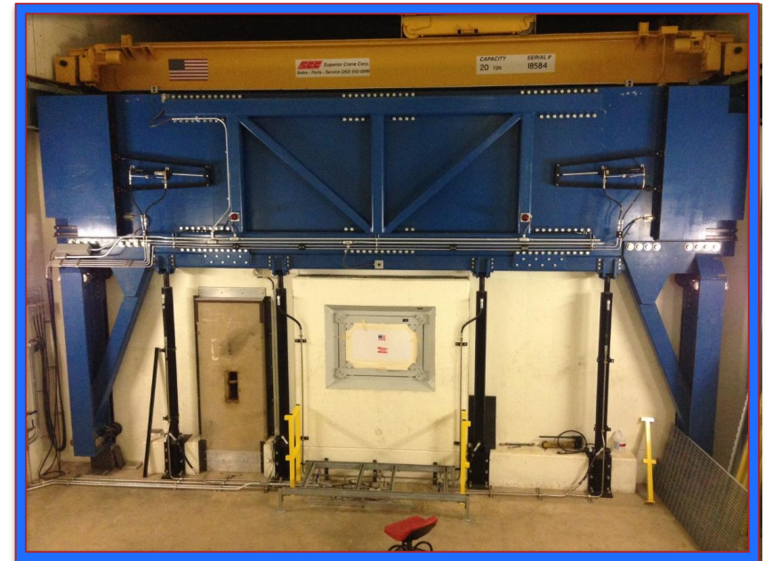
Crane Shield Wall as of 5/28/18
