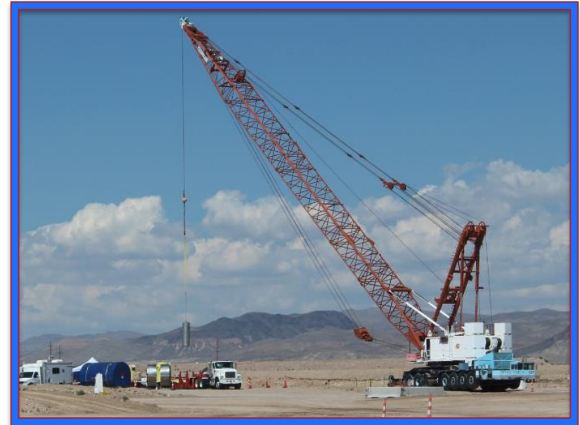
Component Disposal at NNSS
