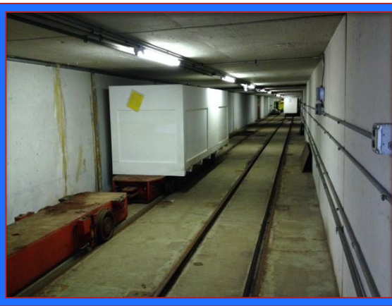
Main Storage Rail Line
