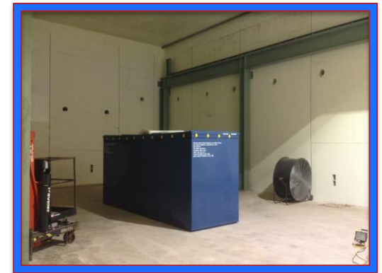
Interior of Hot Bay
