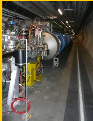
Induced activity monitors
