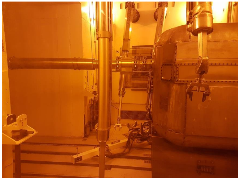
Cross Beam wheeled across the floor and rails.
