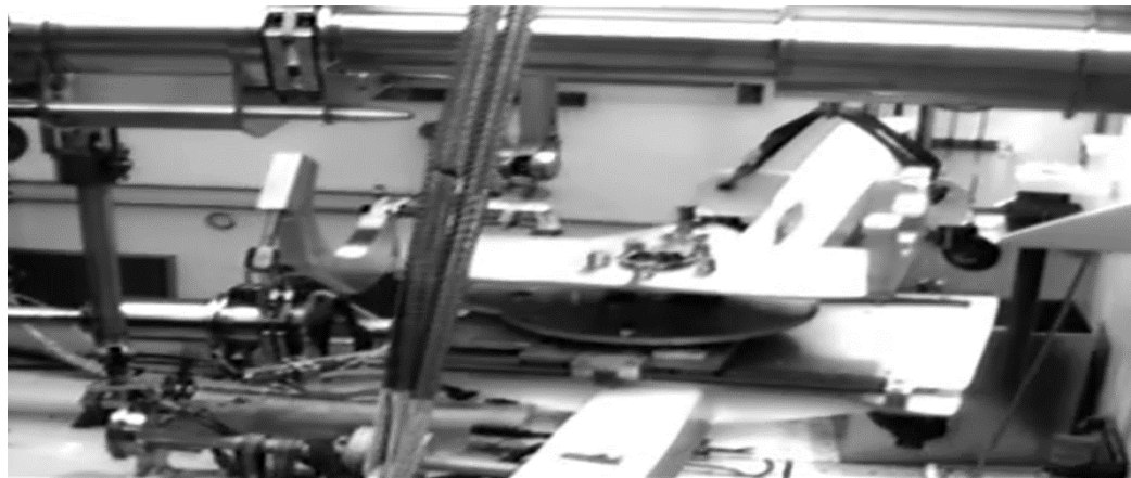
Cross Beam hoisted by crane below the EPB tube
