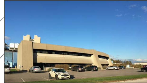
Looking Northeast Towards Booster Tower Southeast
