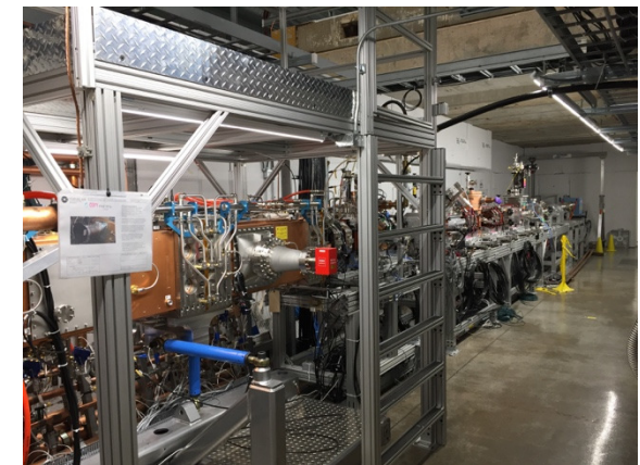
PIP2 Injector Test
