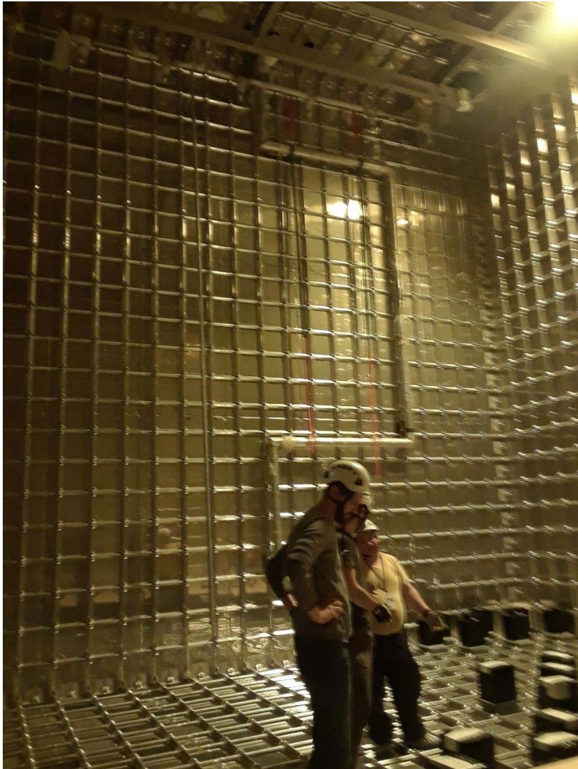
above: completed membrane, false floor & internal cryogenics piping at PDSP; right: Detector support system beams at PDSP
