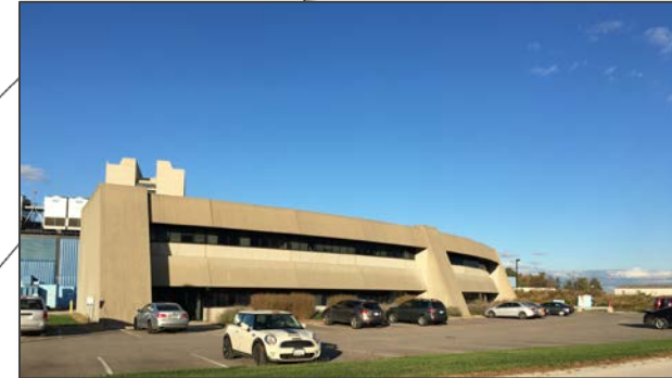
Looking Northeast Towards Booster Tower Southeast
