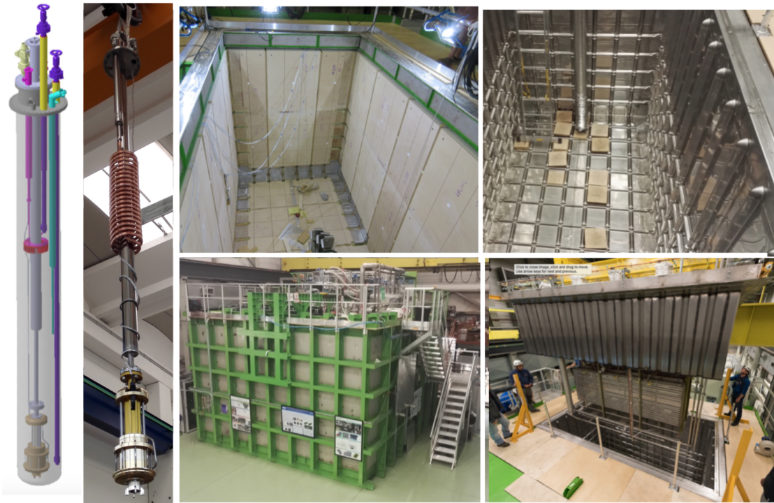
Figure 3: Pictures of the setup at different stages of construction. Left: the pump tower with the extractable liquid pump system. Top: the main vessel interior before and after the welding of the membrane sheets. Bottom right: the top cap with the TPC suspended during insertion in the main vessel. Bottom left: full view of the final cryostat exterior, the cryogenic system is visible on the top.
