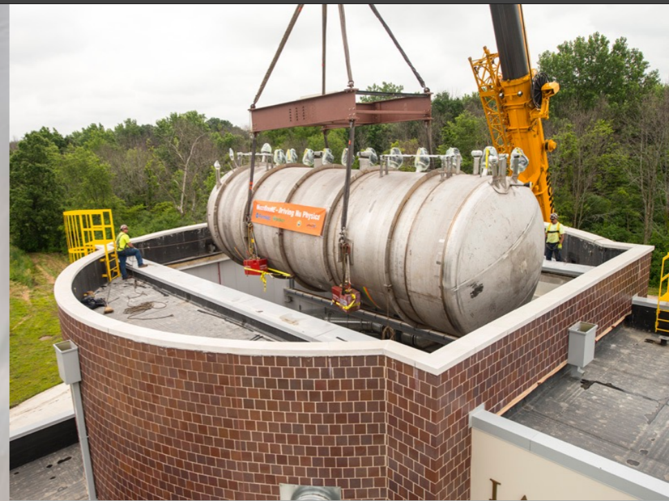
MicroBooNE cryostat lowered into the pit
