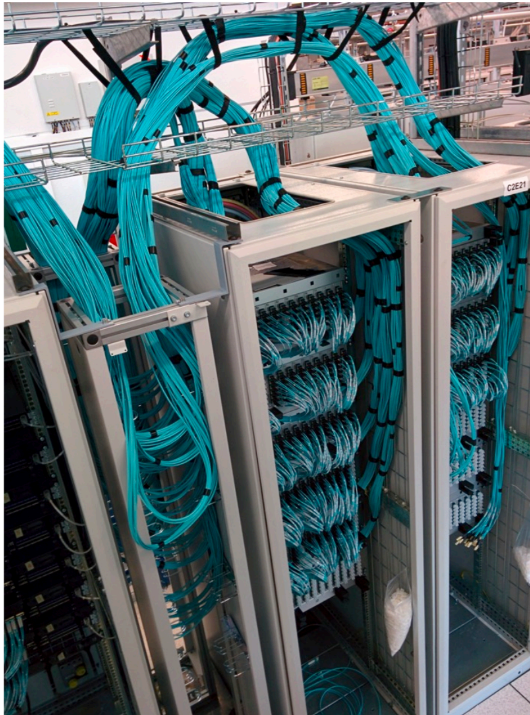
Data concentrator patch panels
