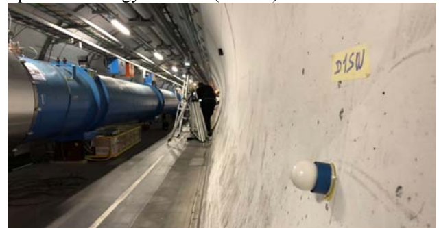
Figure 4 : LHC tunnel with additional network support equipped with a 1.5” white sphere for microtriangulation measurements
