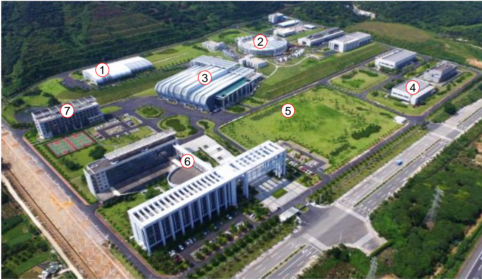
Bird view of CSNS in 2017. Numbering indicates as follows: (1) linear accelerator ; (2) rapid cycling synchrotron; (3) the first target building and experimental hall; (4) main substation; (5) future site of the second target station; (6) office building; (7) service building.
