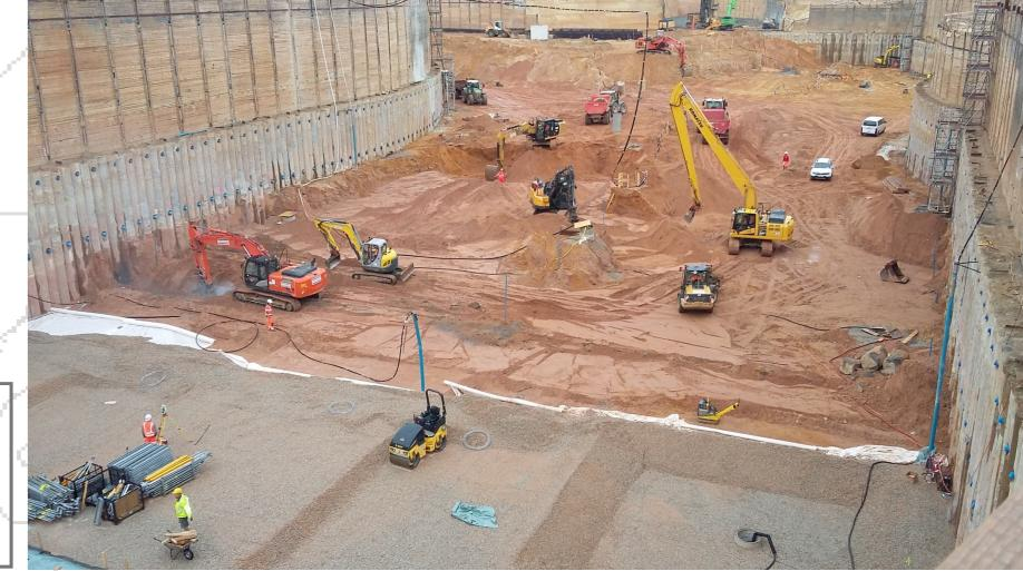
For the construction of the particle accelerator system FAIR, about two million cubic meters of earth must be moved - as much earth as when building a small town with 5000 single-family homes. Around 600,000 cubic meters of concrete and 65,000 tonnes of steel will be used.
