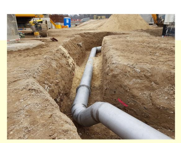
**Approximately 100km pipes for** sewage, fresh water, cooling water, ventilation and electro must be surveyed directly after each placing into the ground before filled up again. 10% of the effort has already been made.
