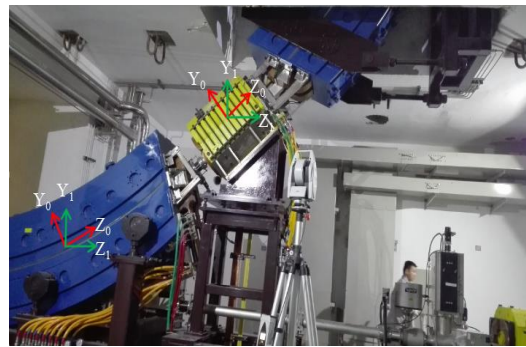
Fig.7 Alignment of high-energy transport lines
