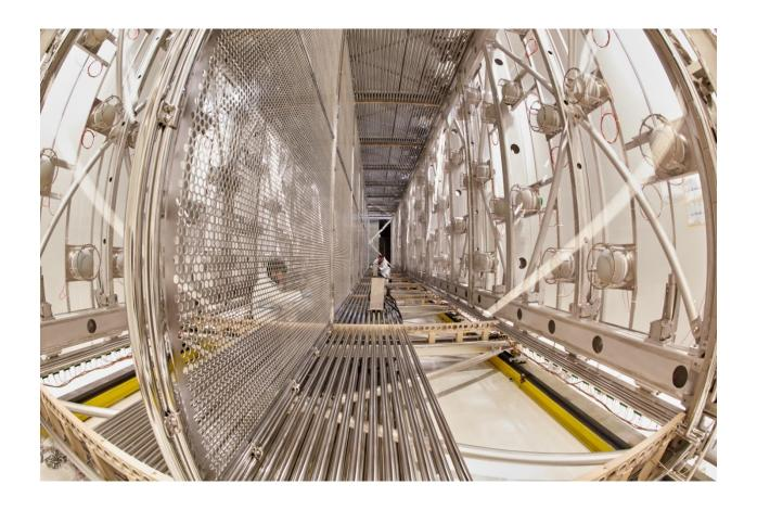
Each cryostat holds liquid argon time projection chamber modules and photodetectors.
