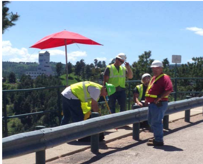
Survey party at the home stake mine utilizing a gyroscope to determine the azimuth between two GPS points
