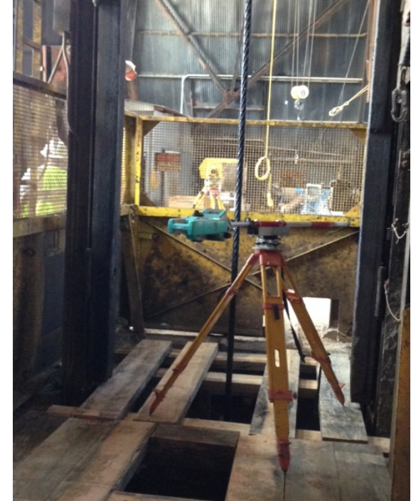
Depth measurement with an electronic distance meter
