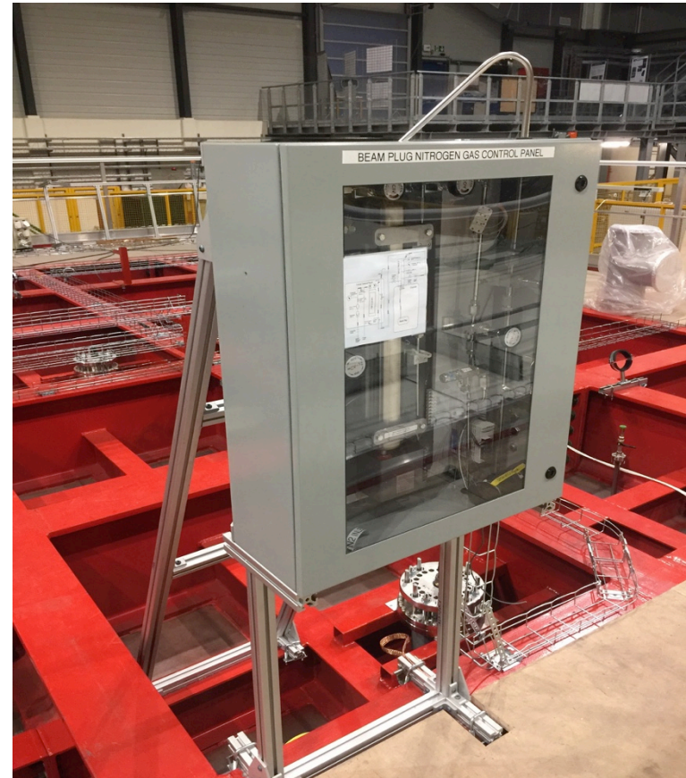
Nitrogen gas controls on top of cryostat
