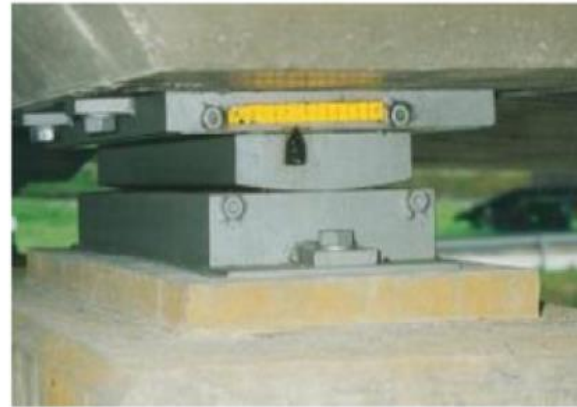
a) Linear rocker bearing
