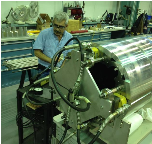
Figure 6.7: Hydraulic rig for pre-tensioning the yoke tie rods.
