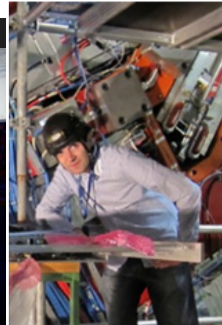
Aram Apyan working on installation
