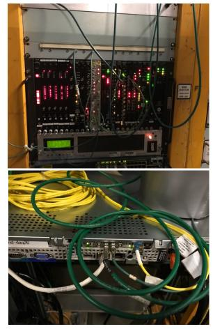
WR node at MI-12 sending BNB beam signals (BES and RWM )
