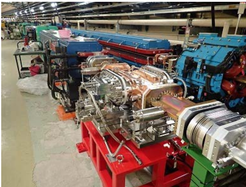
Horizontal type collimator (D02_H1) installed in the tunnel
