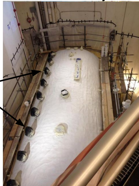
MicroBooNE Foam Insulated Cryostat
