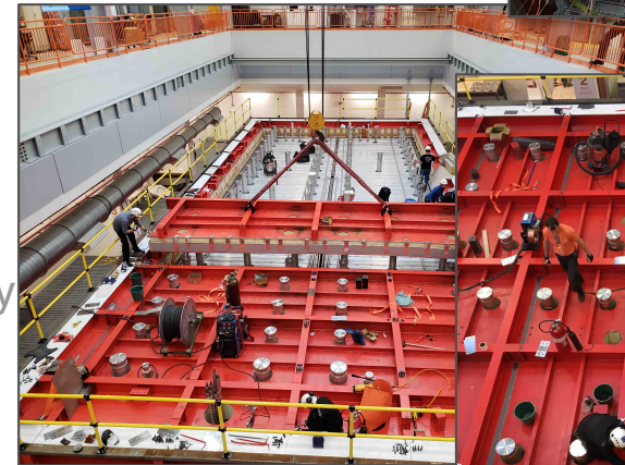
Warm vessel roof installation
