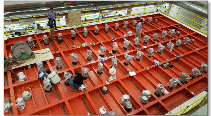
Installing feedthrough crosses
