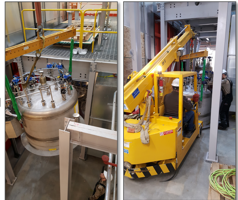
Rigging valve boxes
