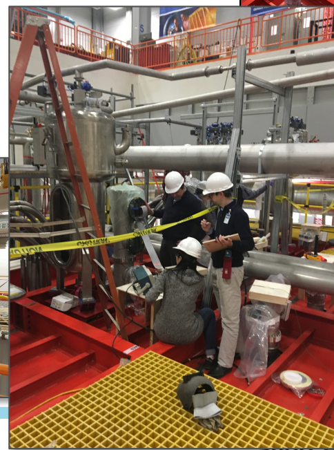
Flange installation and vertical slice test
