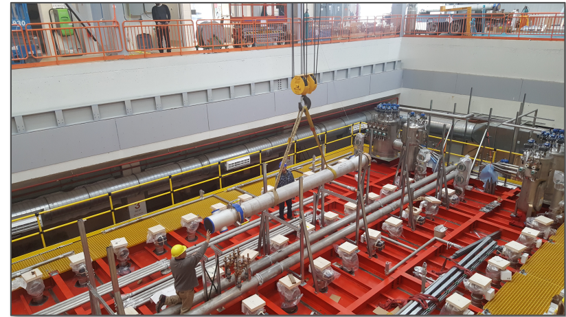
Installing Vent Line (FNAL Scope)
