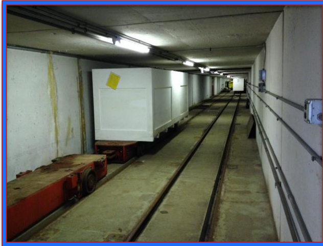
Main Storage Rail Line
