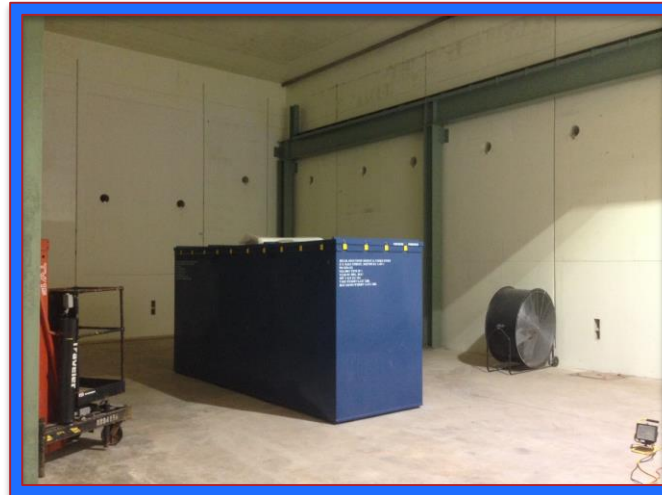
Interior of Hot Bay
