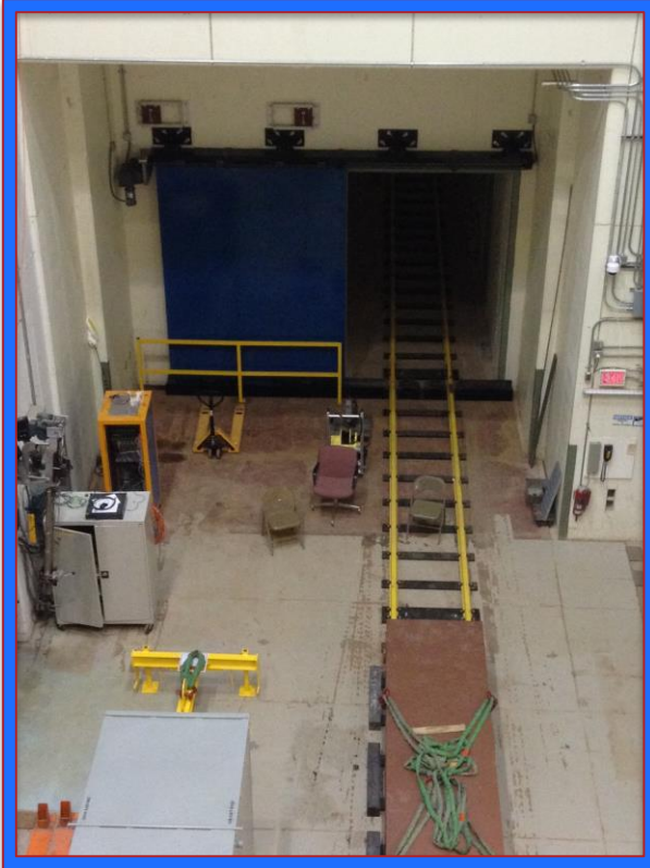
Rail Car & Track 80% Complete
