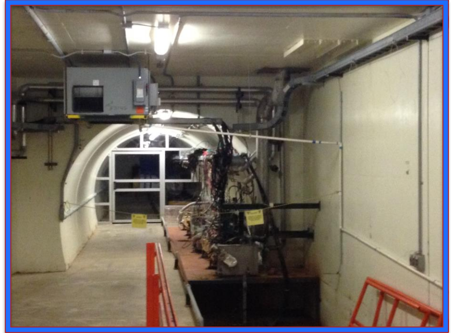
Tunnel Sealing & Dehumidifier Recommissioning 100% Complete
