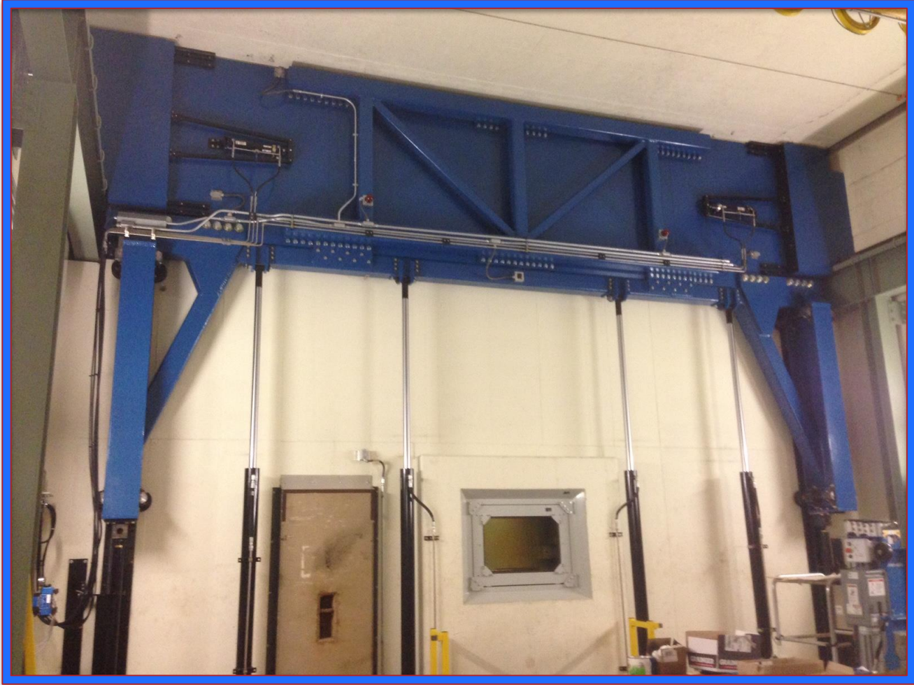
Shield Wall Lifted Into Position
