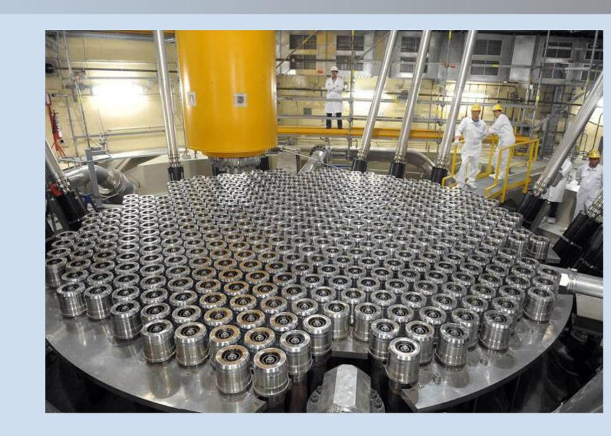
Atucha II is a 2 GW pressurized heavy water reactor located in Argentina,  $\sim 100 \,\mathrm{km}$  away from Buenos Aires. The fuel elements have an active length of 5.3 m. and they are vertically allocated inside a pressure vessel of 8.44 m of diameter. Two positions are being considered, 8 m and 12 m away from the reactor core. They are shielded for most of the background radiation coming from the reactor by concrete walls. For detailed information see poster number 523.
