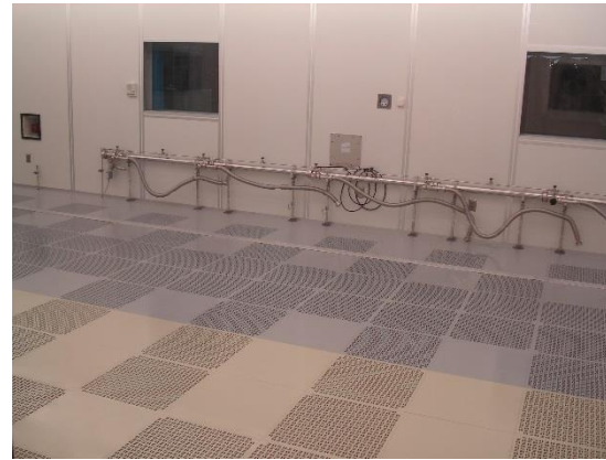
8 stations for pumping, purging and backfilling
