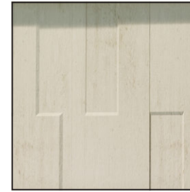
Board Form - Precast Concrete
