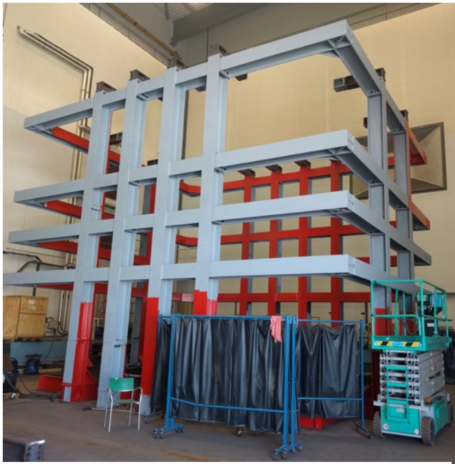
Warm cryostat structure construction at CERN
