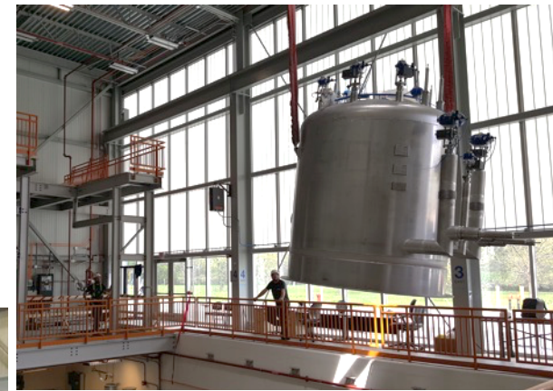
Valve box being craned into position
