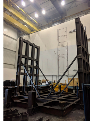
May 28 th Cryostat frame pre-assembly ongoing
