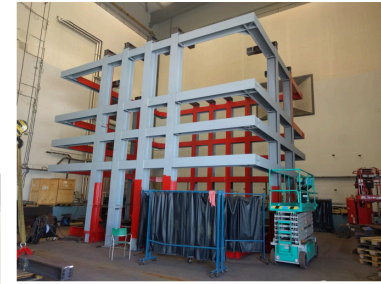
July 10 th Frame pre-assembly and painting near completion
