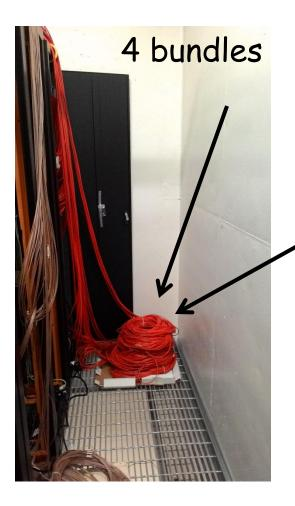
We need to solve the problem of the cable length excess behind the crates on the mezzanine.
